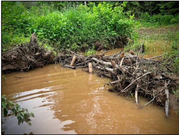
The PALs are slowing the flow of water and allowing sediment to accumulate behind the structures as intended.
