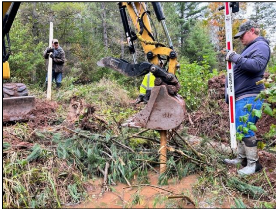
Light equipment was needed for PALS installation in dense clay soils.
