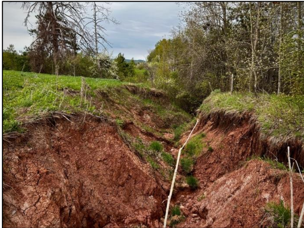
Severe gully encroaching into the cropped fields on the Berweger Farm.
