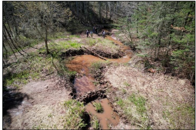
Aerial image of two installed PALS at the Tody Ravine. Bank incision visible on outward bend. (Credit: Trout Unlimited)
